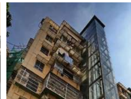
Modernization and Upgrading
